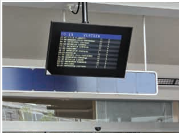
Saint Nicolas Station / Belgium
